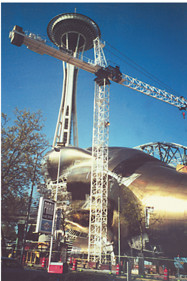
Challenging Construction Management project
